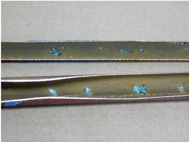
Figure A.3 – Pipe C
