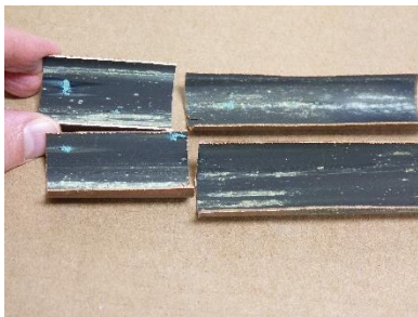
Figure A.5 – Pipe F
