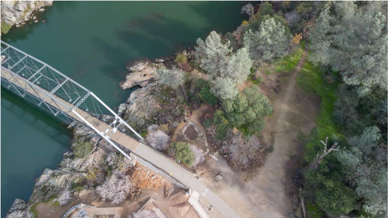
View of the Historic Truss Bridge and existing river overlook area from above
