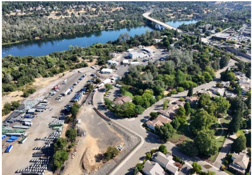
The central plan segment includes the Corporation Yard (foreground) and the Historic District
