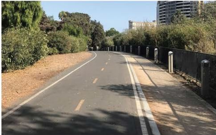
A soft-surface shoulder alongside a shared use path provides additional space for trail users, particularly runners or others who prefer natural surface trails.
