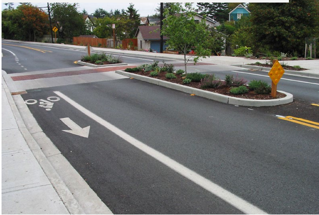
Median Refuge Island, Raised Crosswalks
