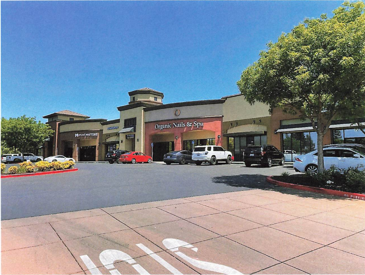
FIGURE 1: FOLSOM DAM RETAIL SHOPPING CENTER
