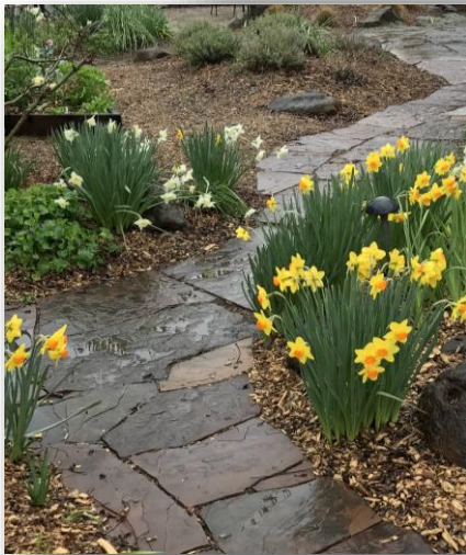
Flagstone with gravel joints
