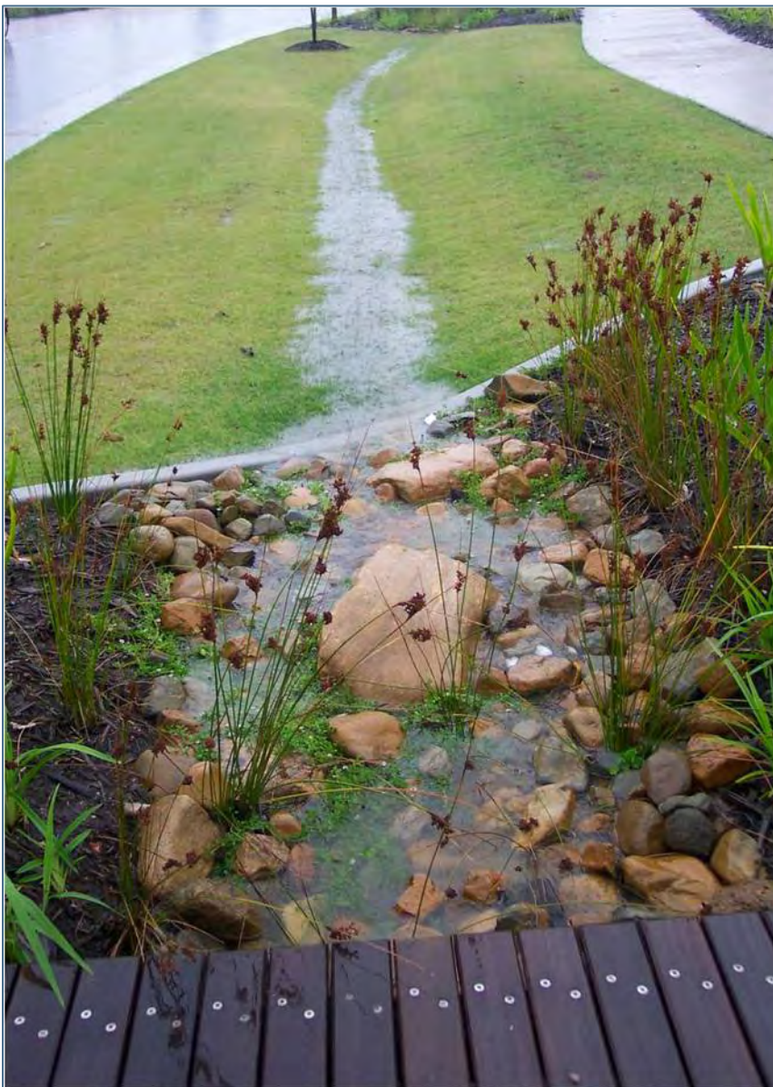
Vegetated swales and drainages are generally the recommended design for conveying stormwater runoff to the creek.
