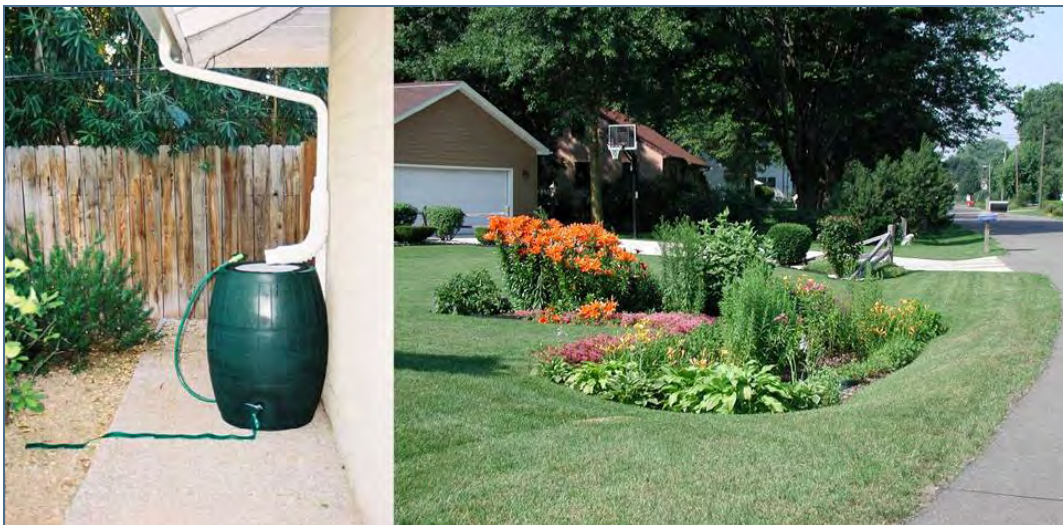
Examples of small-scale stormwater systems in residential lots using rainwater barrel and rain garden.
