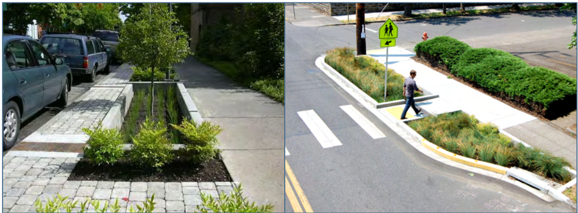
Examples of curbless street and street with regular curb-cuts to allow stormwater to flow from streets into the infiltration areas.
