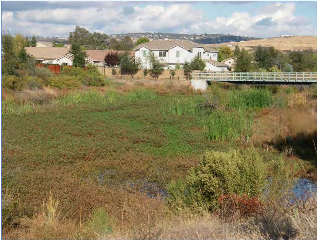
Detention basin on the north side of U.S. 50 with extensive stands of nuisance aquatic vegetation.
