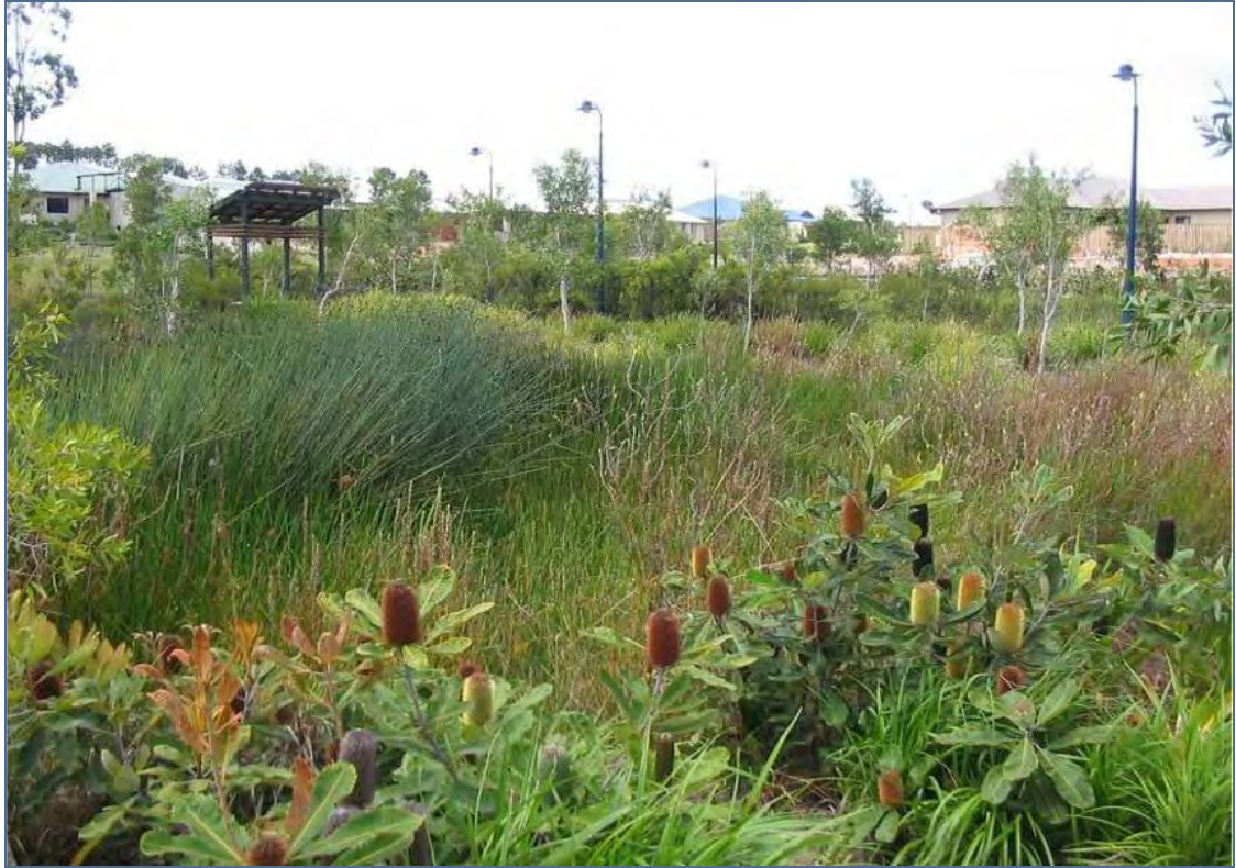
Stormwater detention basins vegetated with wetland species provide multiple benefits, such as wildlife habitat, water quality improvement, and visual interest.
