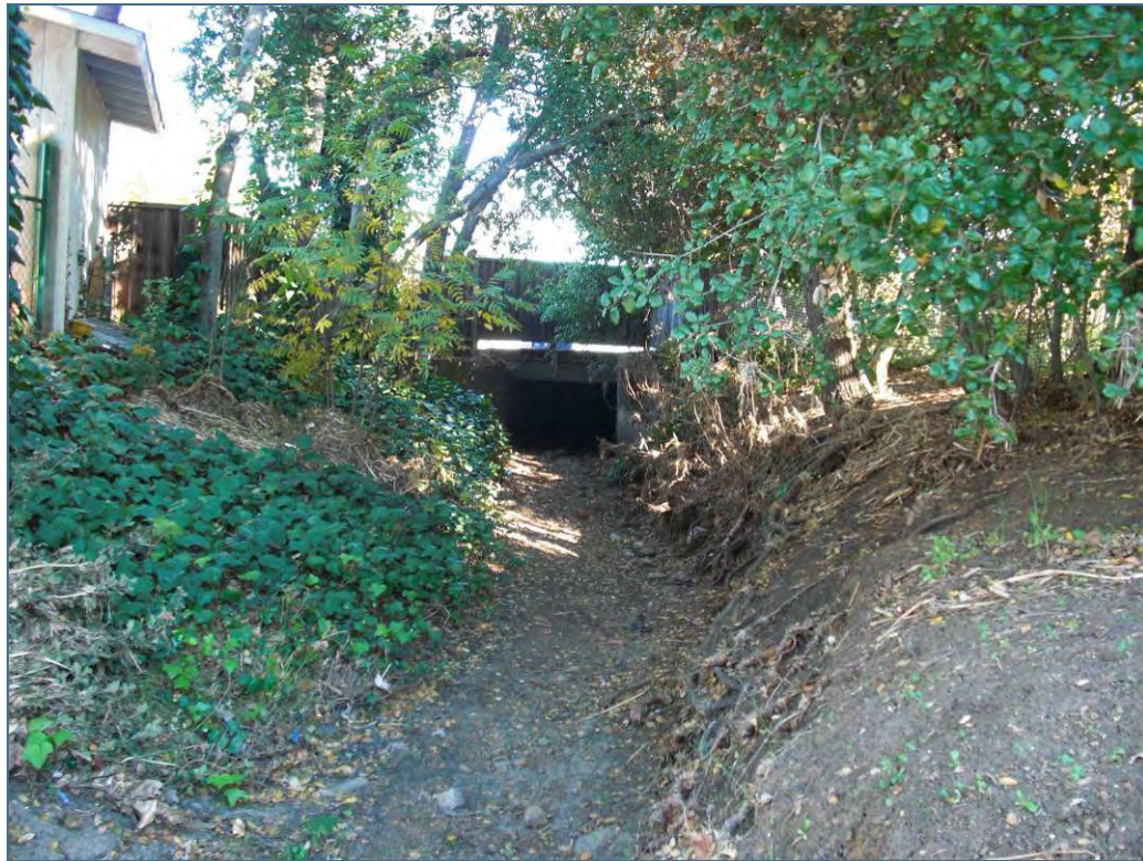
Bottomless box culverts provide sediment transport and movement benefits that piped culverts do not.
