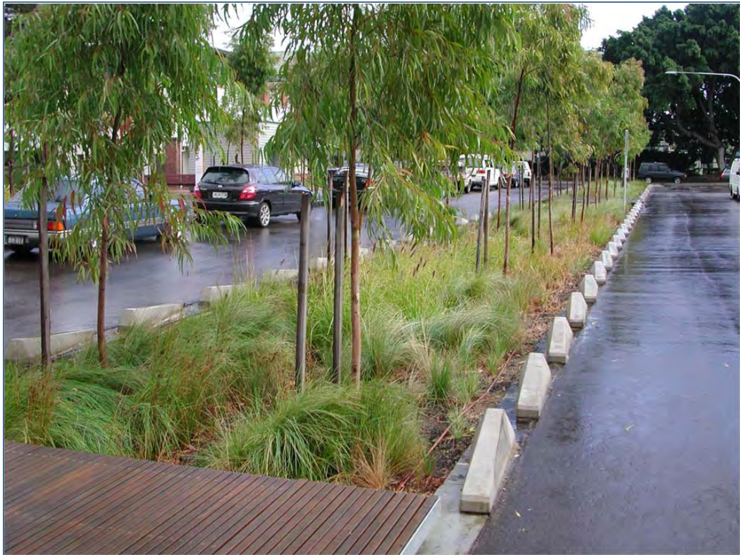
Small biofiltration systems integrated with entrance landscaping, front setback of corner lots, parking bulbouts, and landscaped medians.
