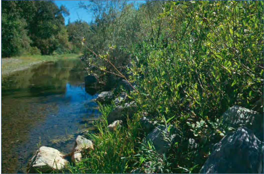
Vegetated riprap provides bank stability and habitat.
