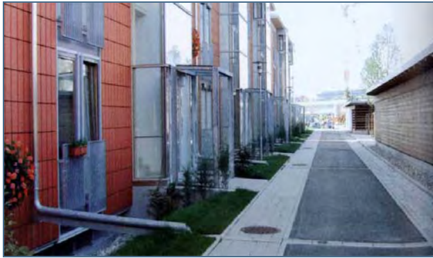
Using disconnected roof drain to channel water to vegetated area and pervious pavement.
