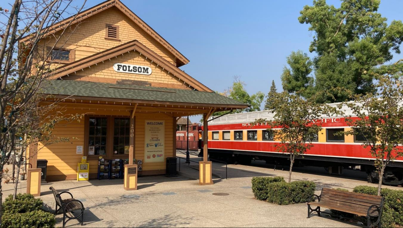
Southern Pacific Railroad - Folsom Depot Building
