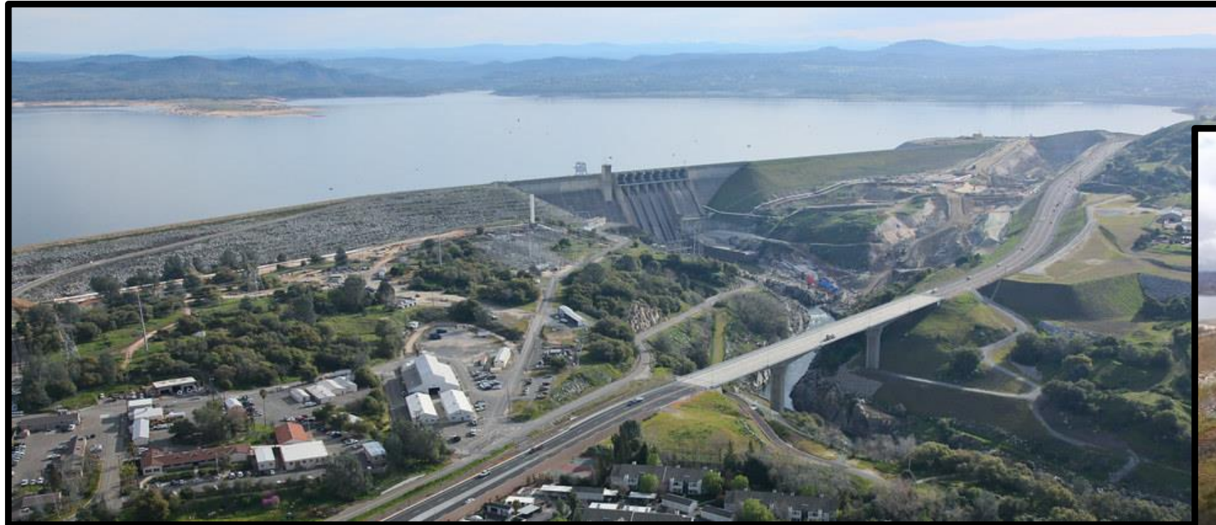
Folsom Dam Raise Project
