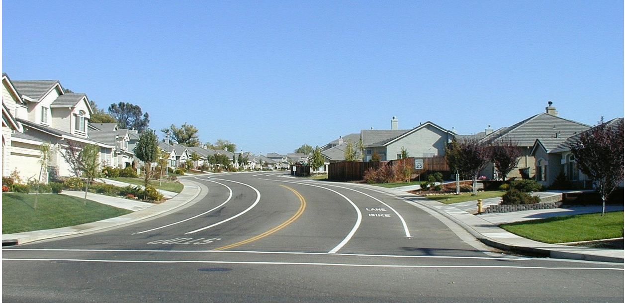
Bike lane striping used for traffic calming along Lembi Drive.
