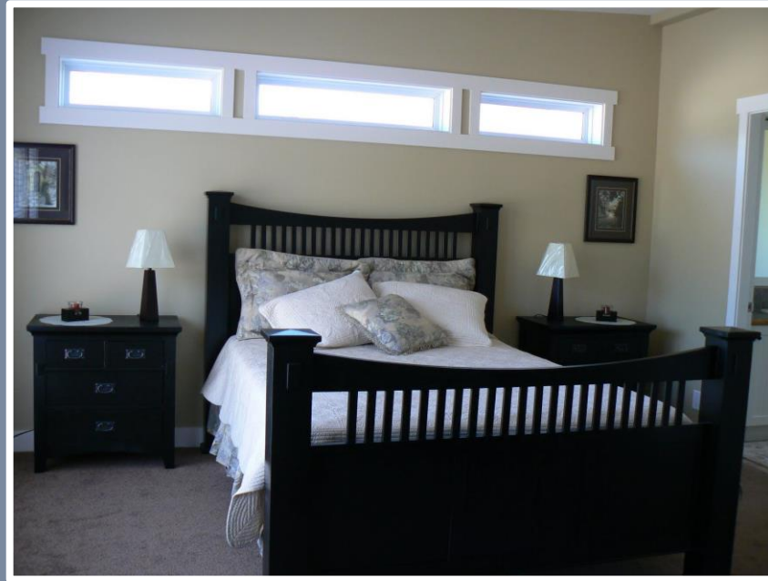
Use of clerestory window in 2 nd floor bedroom allows for natural lighting but protects the privacy of neighbors.
