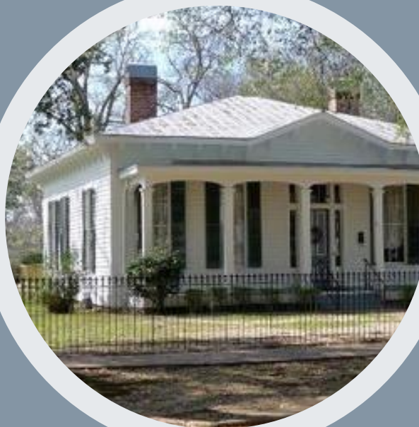
Single-story porch with hipped roof and paneled door
