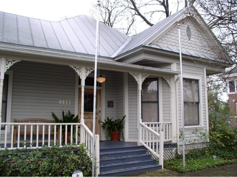
Porch with spindlework
