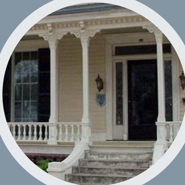
Single-story porch with horizontal wood siding and paneled door
