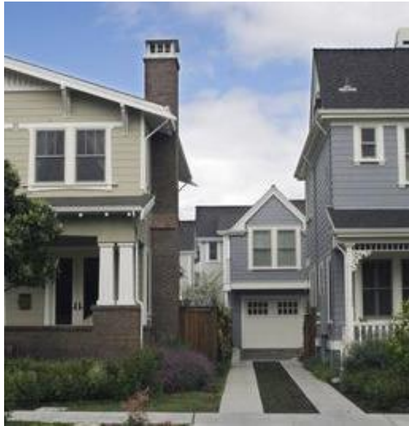
Detached two-story ADU designed to match primary home. Notice the use of similar siding, trim, and roof pitch.
