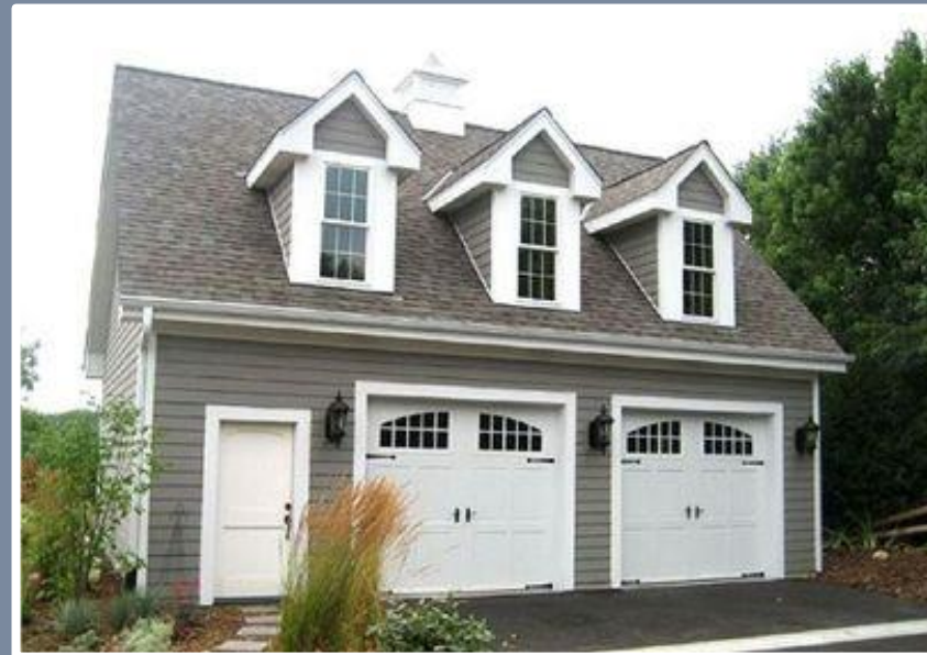
Internal staircases help maintain privacy of adjacent properties.
