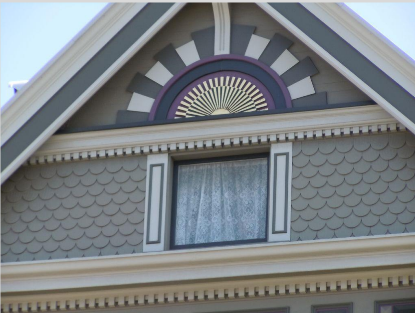
Scalloped shingles with window at end of forward-facing gable
