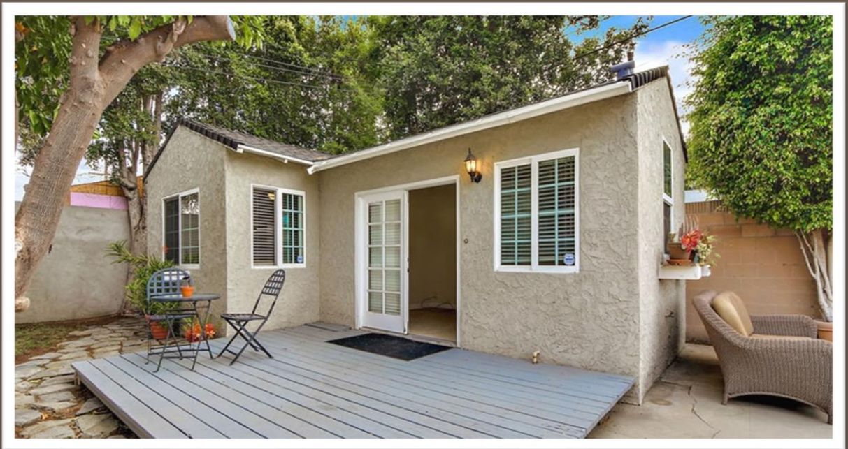
Low roof pitch with lack of decorative wall detailing
