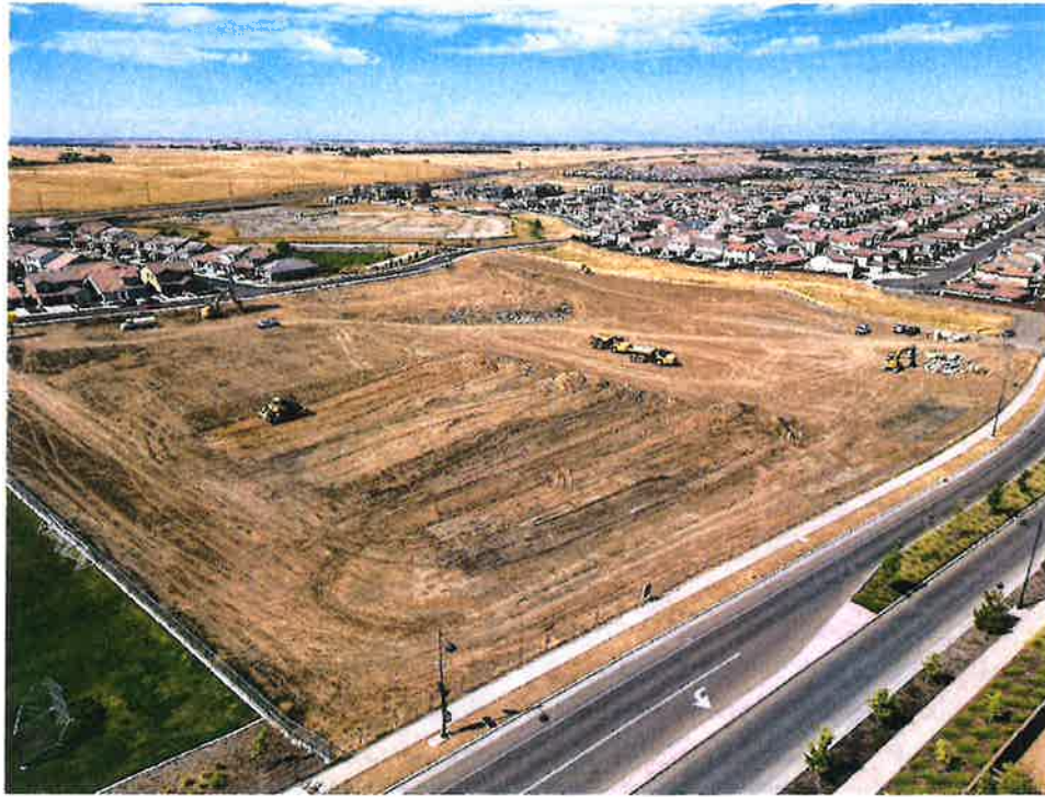
Prospecter Park Rough Grading
