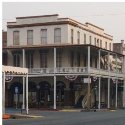
REFERENCE - 3 STORY BLDG. - OLD SACRAMENTO
