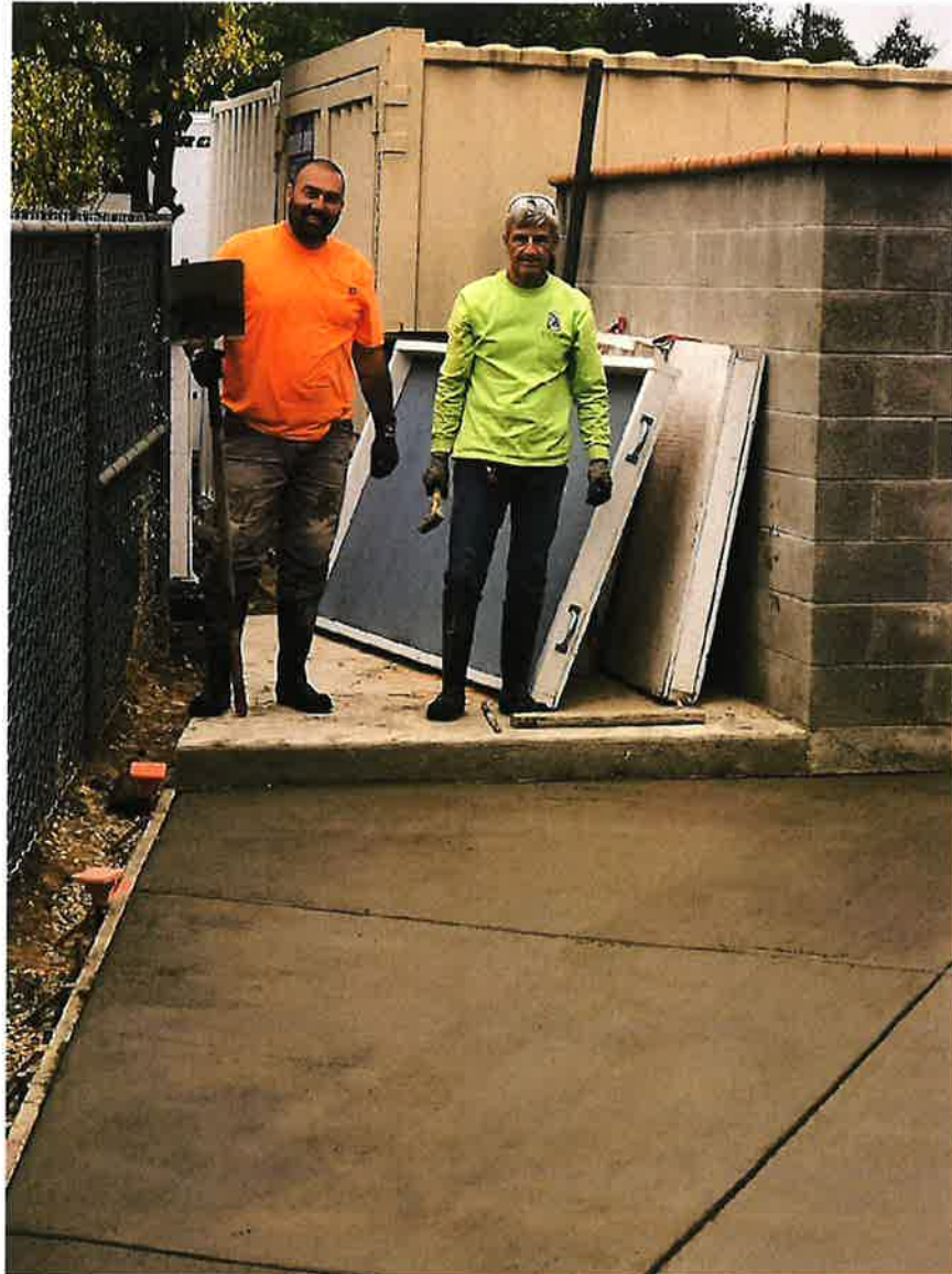
Concrete Installation at Fire Station 35
