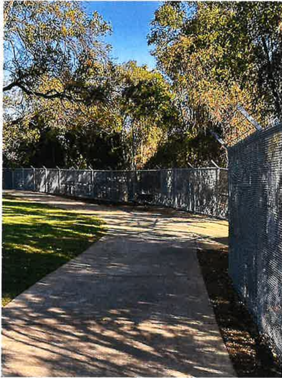
New Zoo Perimeter Fence
