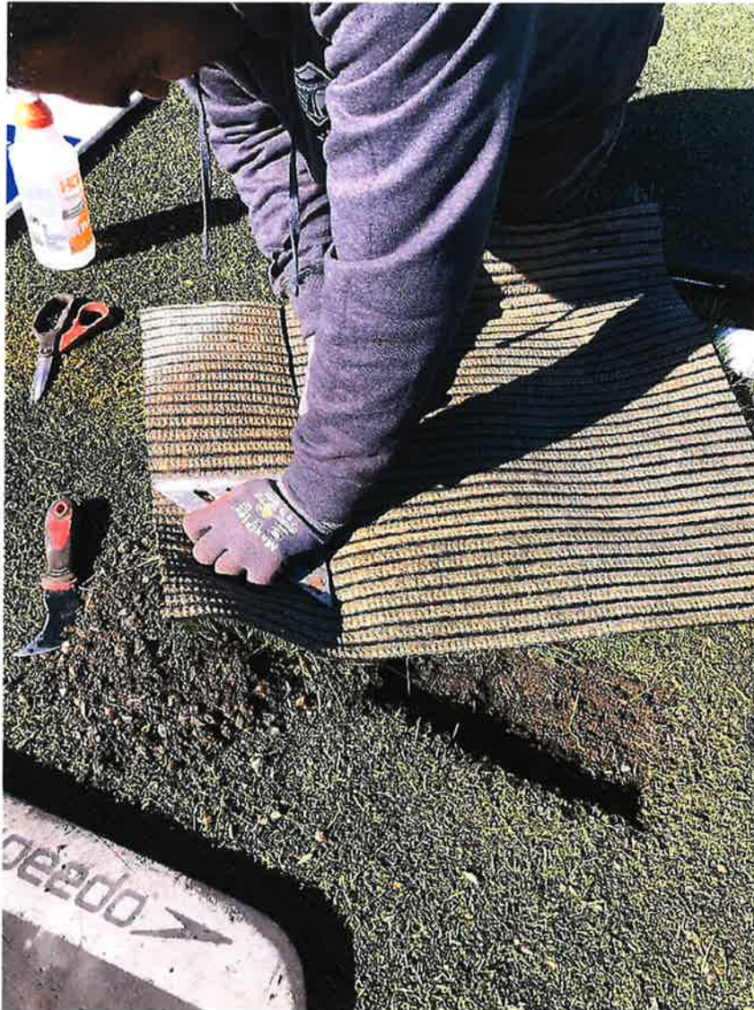
Artificial Turf Repair at Kemp Park
