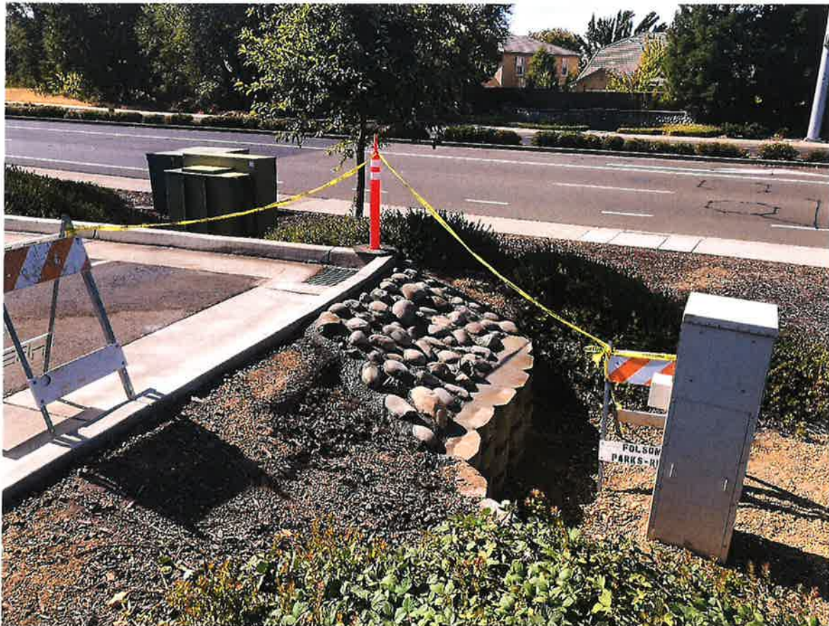
Slope Repair at Broder Parking Lot
