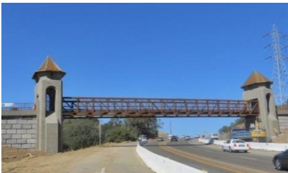
Some communities use arches or highly visible signage to signify a community gateway. The Johnny Cash Bridge serves as a gateway into Folsom.
