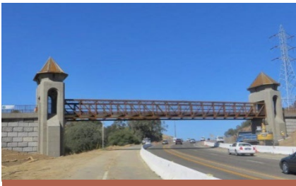
Some communities use arches or highly visible signage to signify a community gateway. The Johnny Cash Bridge serves as a gateway into Folsom.
