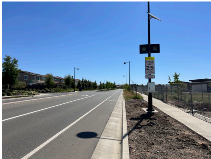
The existing school zone warning lights
