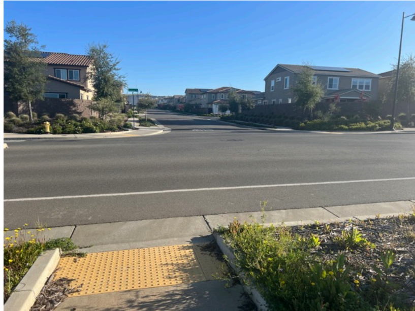
Mangini Pkwy and Wildflower Way Intersection
