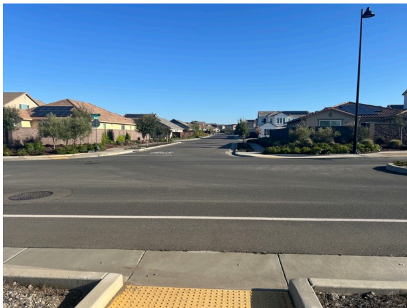
Mangini Pkwy and Rock Hearth Dr Intersection
