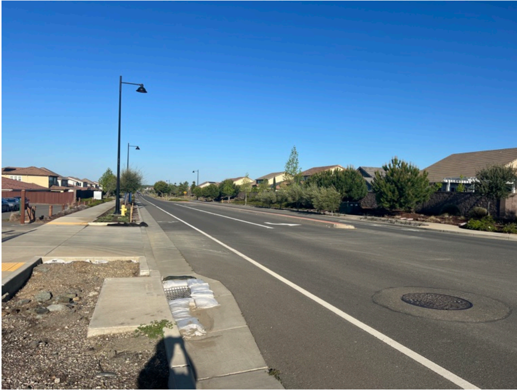
The view of west from the eastbound Mangini Pkwy (Wide on-ramp to the park shown)
