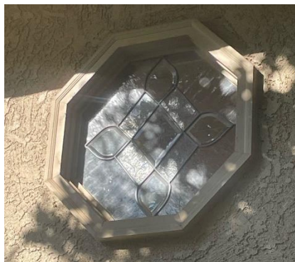
Figure 1 – Existing Octagonal Window
