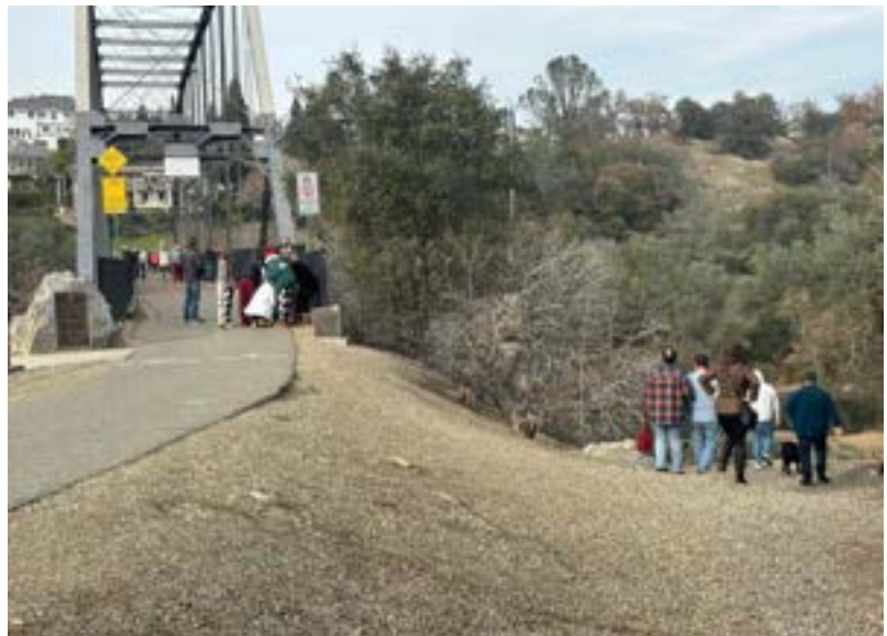
The area around the Truss Bridge is frequently congested with a multitude of trail users and people seeking access to the water
