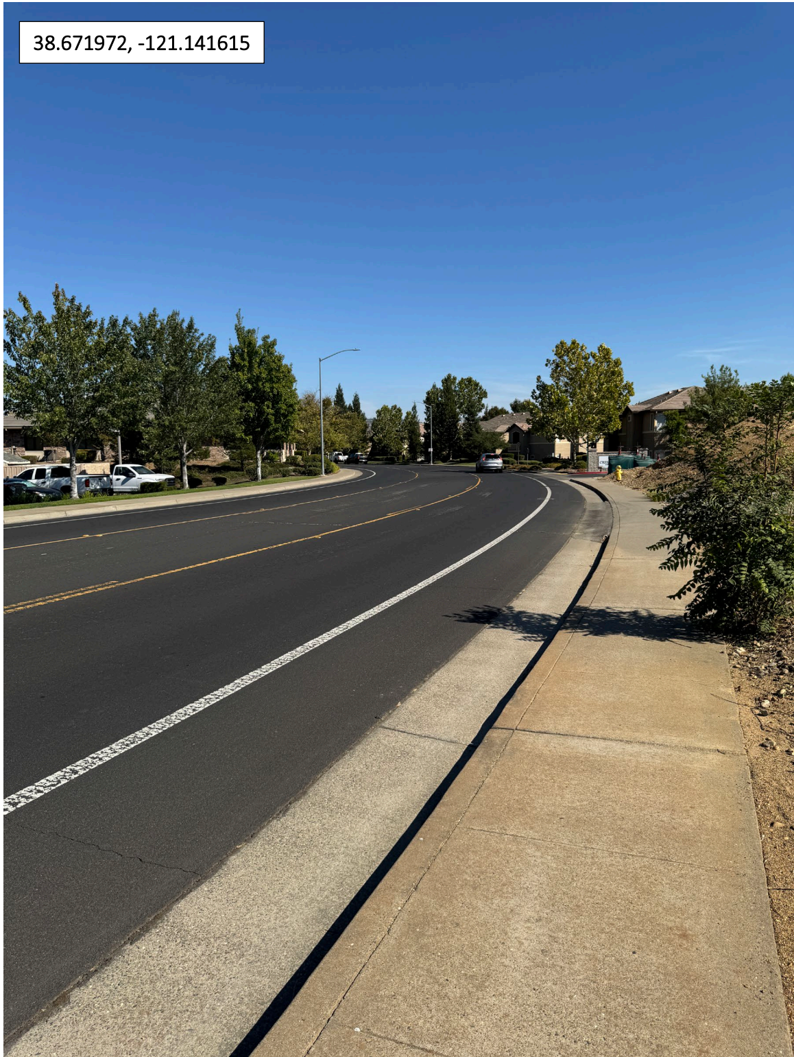
Figure 2 – Creekside Drive (~150 ft west of Creekview Manor driveway)
