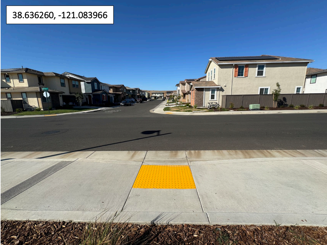
Figure 2 - Existing Conditions (Harvest Gate Wy)
