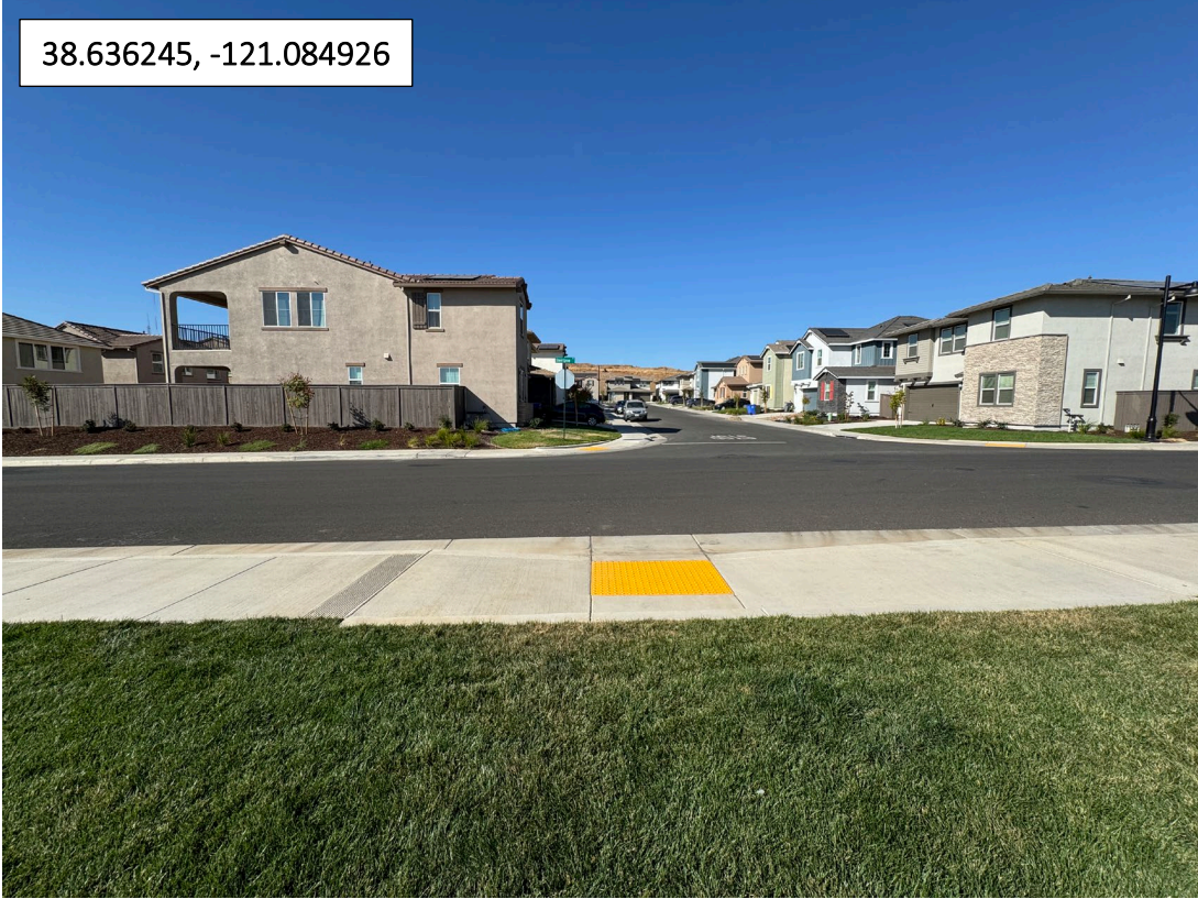
Figure 3 - Existing Conditions (Via Rancho Wy)
