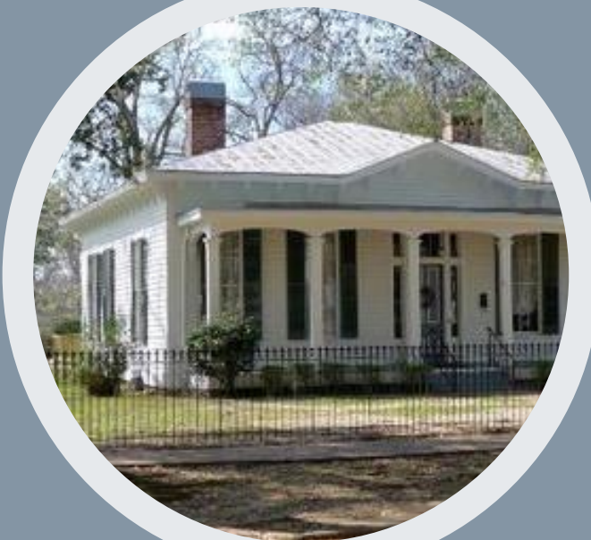
Single-story porch with hipped roof and paneled door
