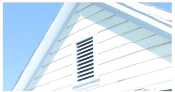
Simple rectangular gable-end vent
