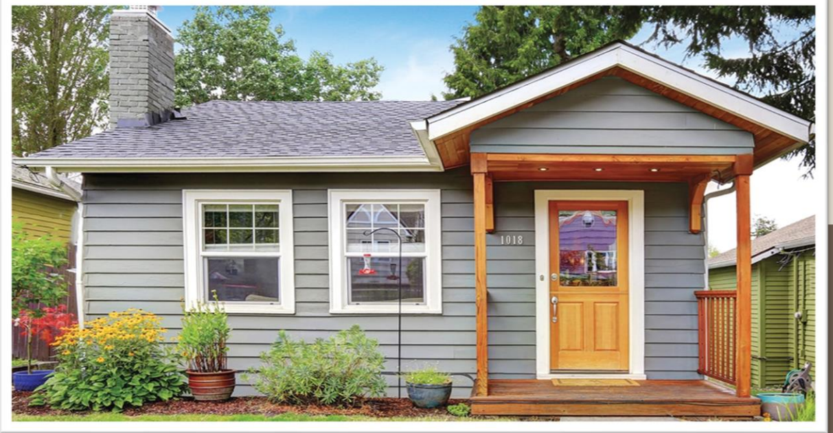
Front-facing gable with soffited eaves
