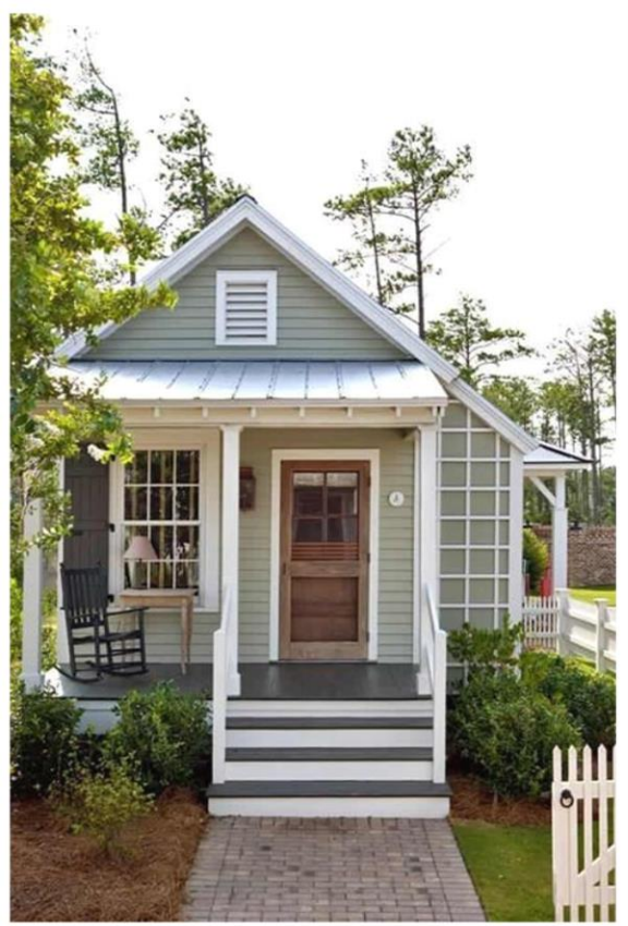
Low-pitched roof over porch
