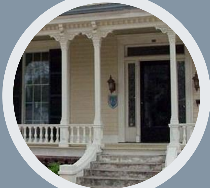
Single-story porch with horizontal wood siding and paneled door
