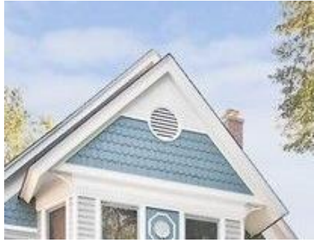
Scalloped scale shingles with vent at end of forward-facing gable
