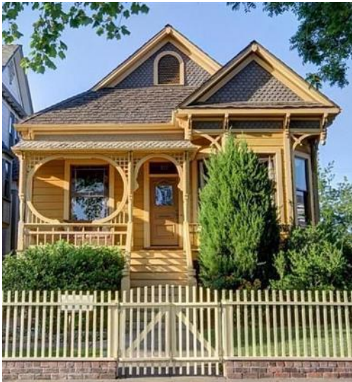
High pitched hipped roof with cross gables
