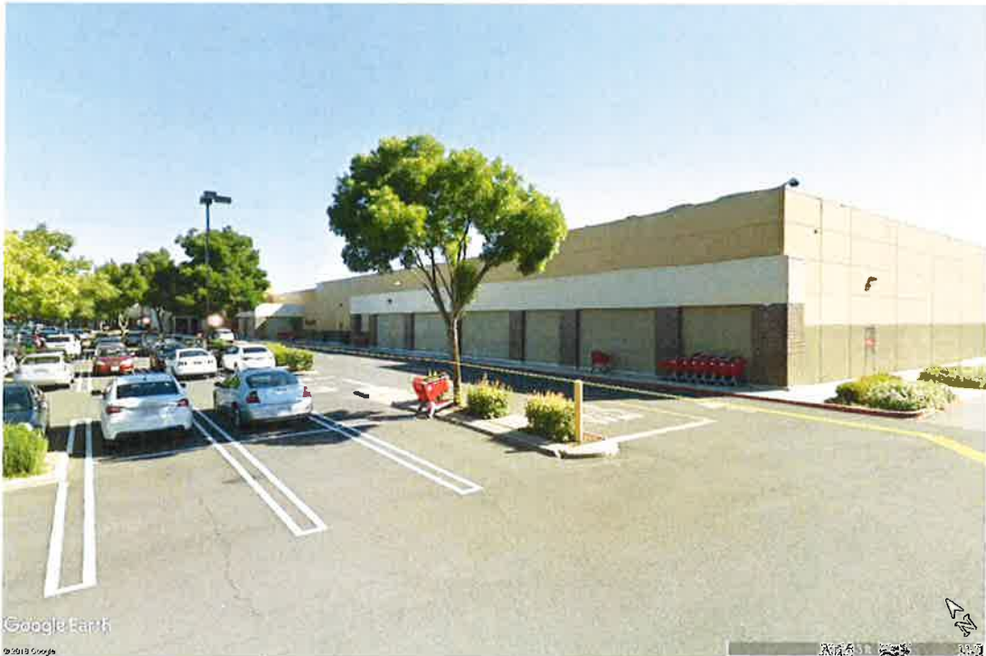
Photo 4: View of southern corner of building facing north.
