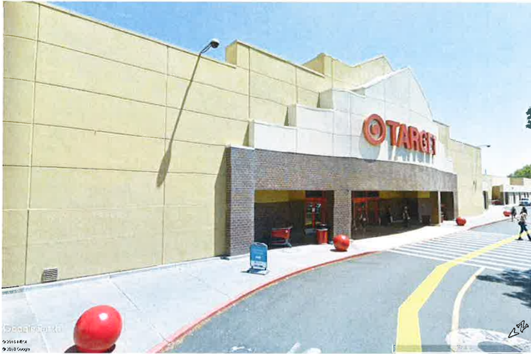
Photo 1: View of storefront entrance facing south.
