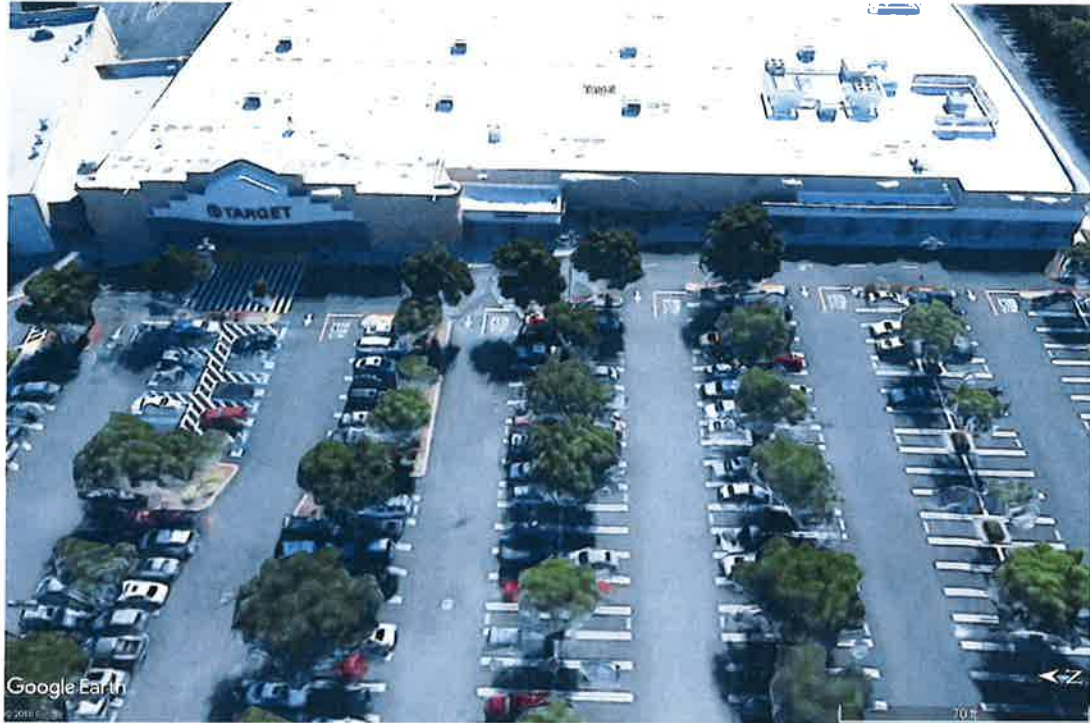
Photo 5: Aerial view of store facing east.
