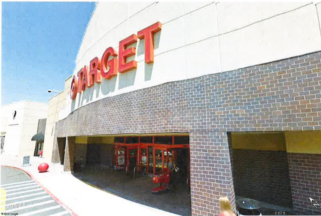
Photo 2: View of storefront entrance facing north.
