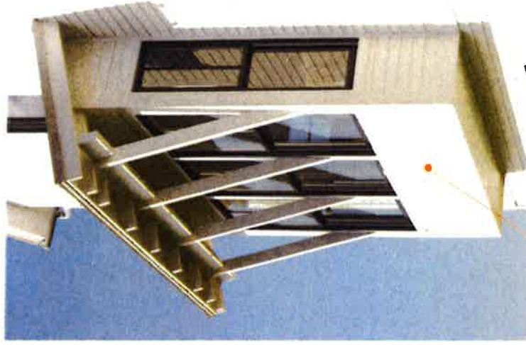
Room and porch dormers with open rafter tails under shed roof
