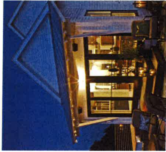
Porch post corbels and entry door side-light windows
