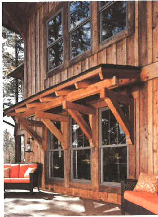
Corner key construction
