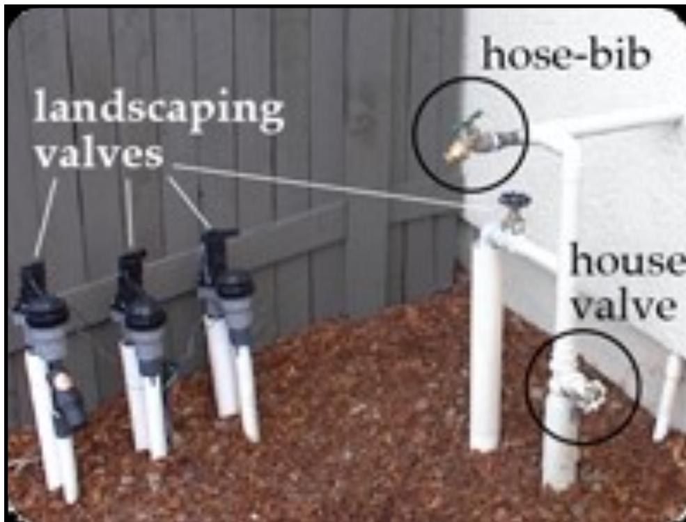
**Inspect areas around the valves or valve manifold for leaks and/or pooling water.**
