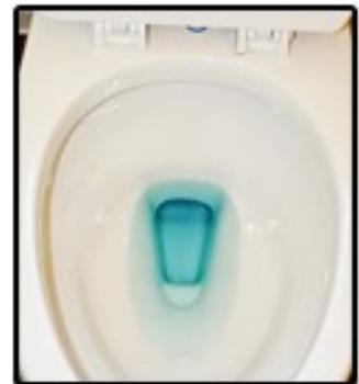
Wait five minutes and check to see if any coloration appears in the toilet bowl. If the water in the bowl has changed color, the problem is either a leaking flapper valve or the flapper chain needs to be adjusted.
