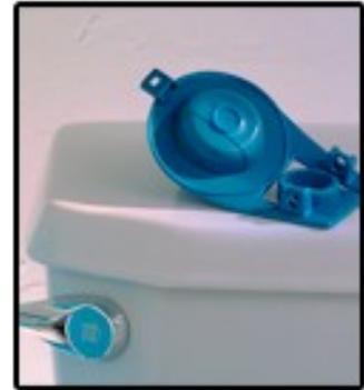
To determine if this is your problem, conduct a dye test using leak detection dye tablets or food coloring.
