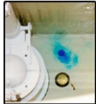
Place the dye tablets or coloring agent in the tank. The water in the tank should change color, but the water in the toilet bowl should remain clear.
