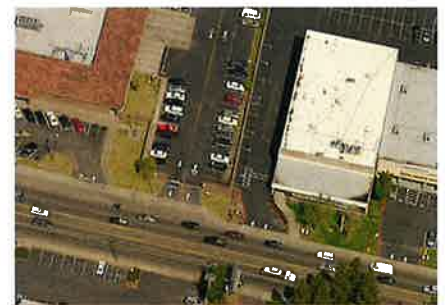
These two strip malls in another community have four driveways nearly adjacent to each other. This creates an unsafe and unpleasant environment for pedestrians and drivers.
