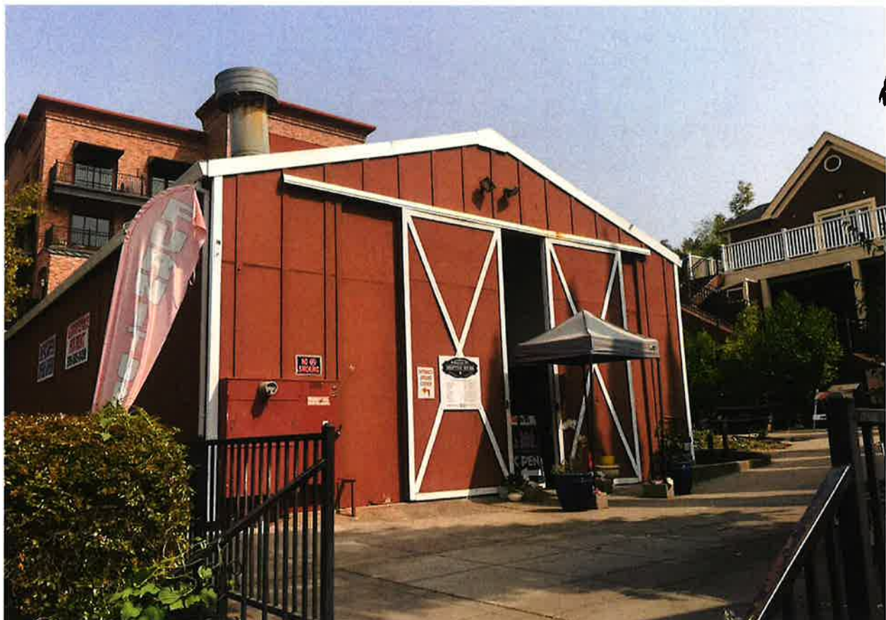
FIGURE 4: COMMERCIAL BUILDING AT 608 ½ SUTTER STREET
