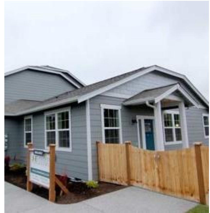
Attached ADU with separate entry that matches original home using same color, trim, horizontal siding, and roof shingles.
